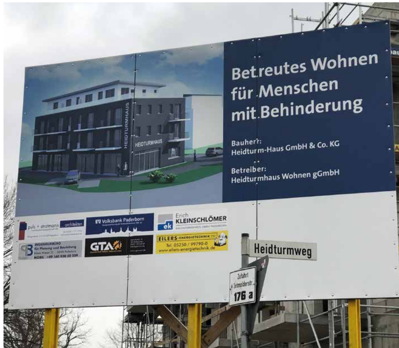
House for assisted living for people with disabilities, Heidturmweg, Paderborn, Germany
